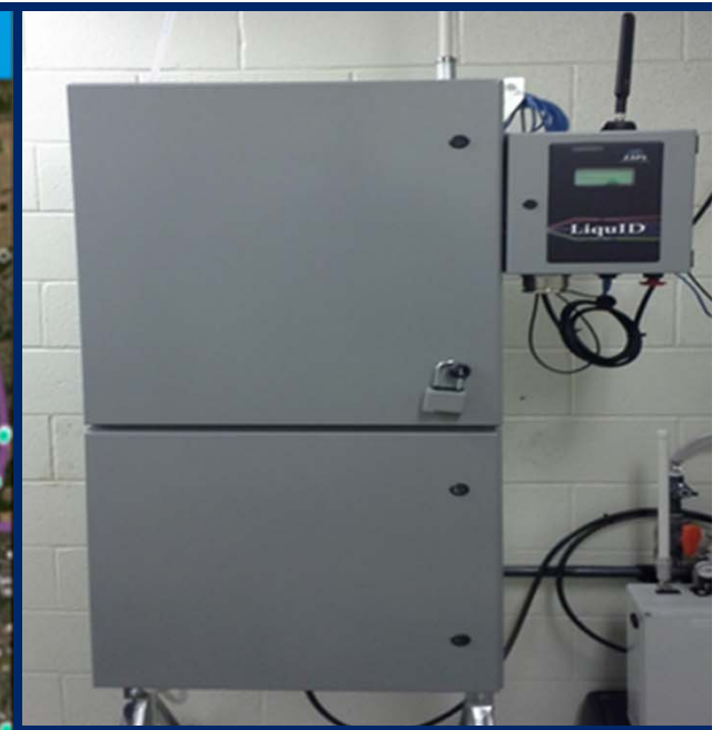
In-stream toxicity sensor
